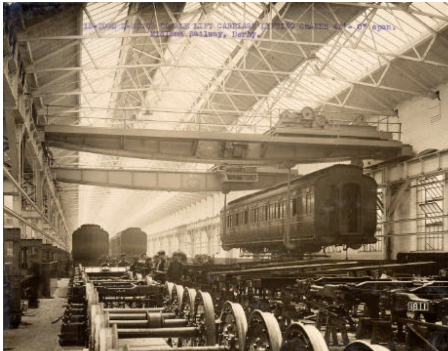
One of Craven Brothers cranes being used to move carriages for the Midland Railway, Derby.
