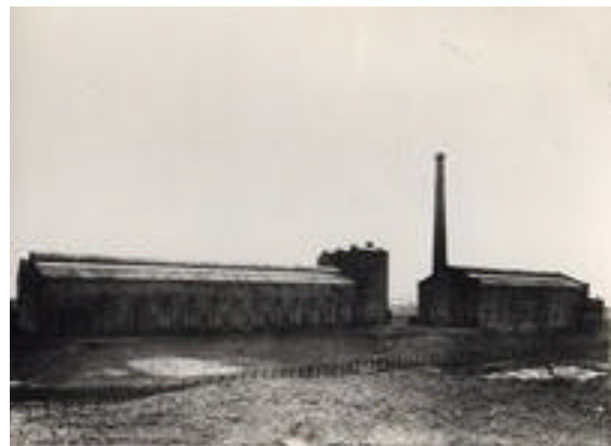
The Hollinwood factory.
